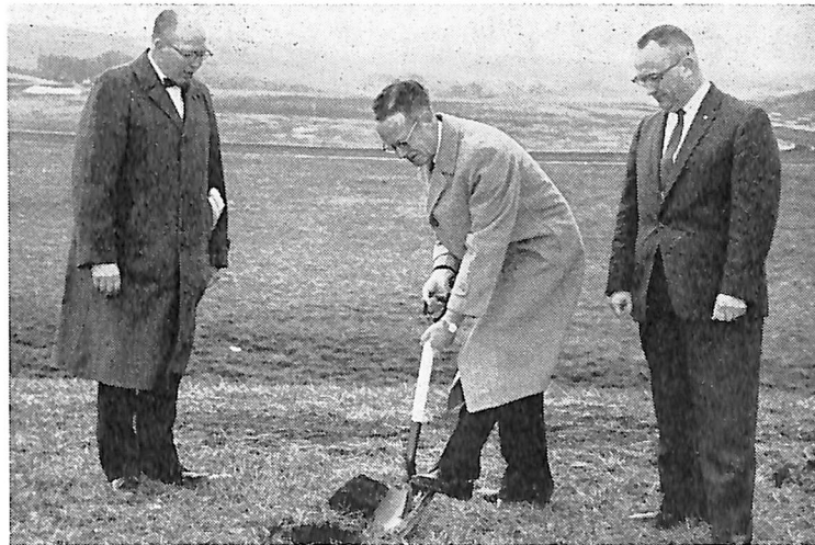
At ground breaking . . . (from left) Olsen, Dr. Madsen and Krantz
