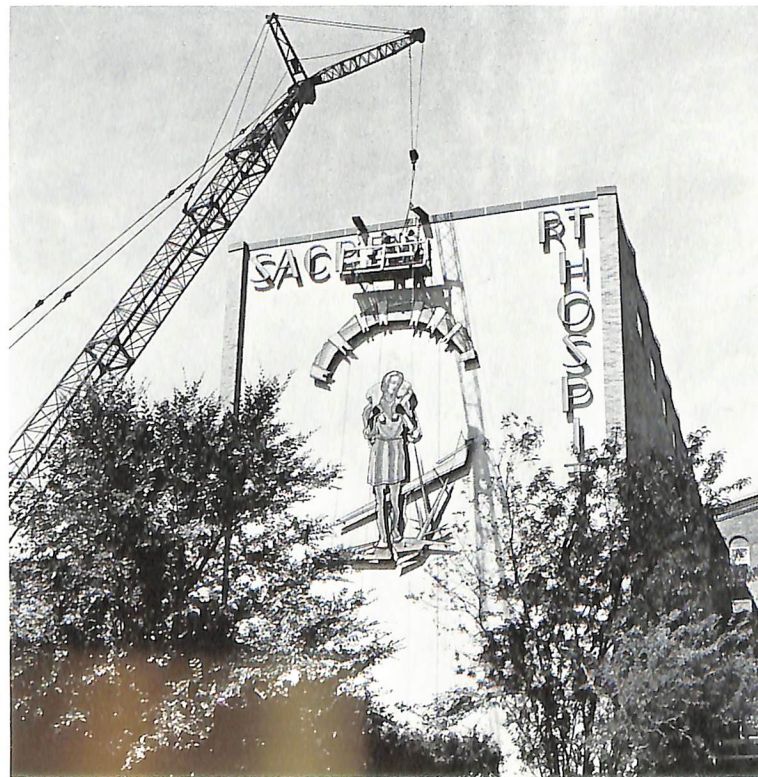
Finished work (left). Giant crane hoists it into position (above). (Photos by James Denney)
