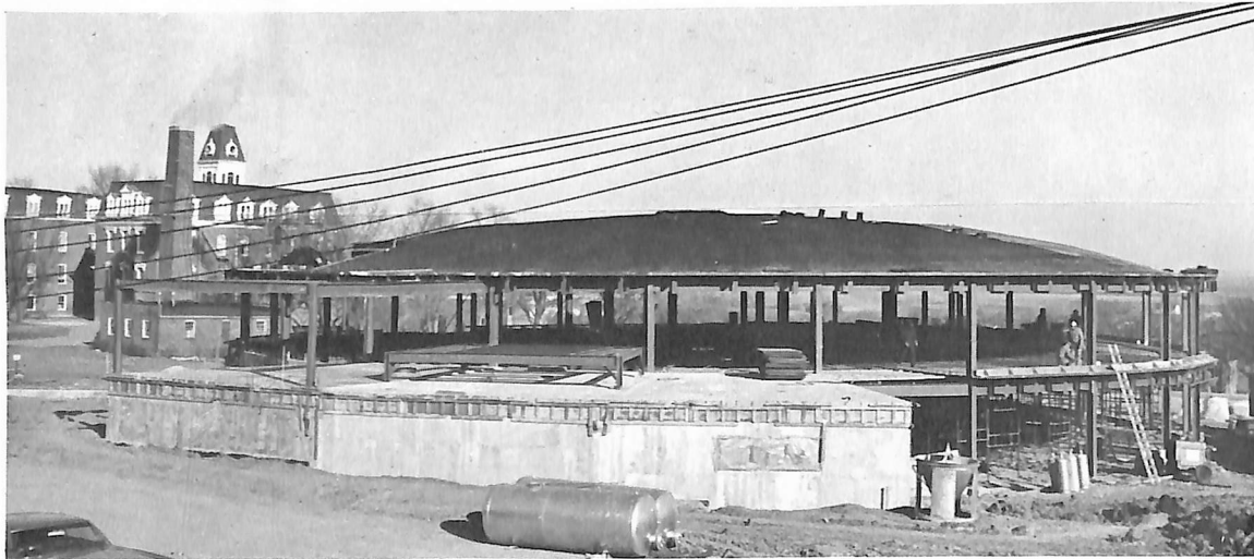
Campus Center Shows Its Ribs, Soon To Be Covered
