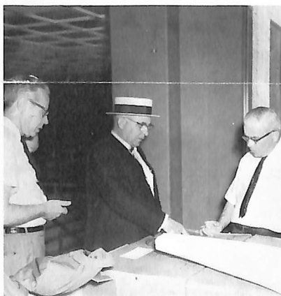
Will they be finished in time? Quite possibly that was the question asked by President Madsen (left) and Business Manager Snowbeck (right) as they met for an impromptu conference with Head Contractor Simon Korshoj, president of the Korshoj Construction Co. The camera caught this unposed shot following the initial placement of books in the new Library.
