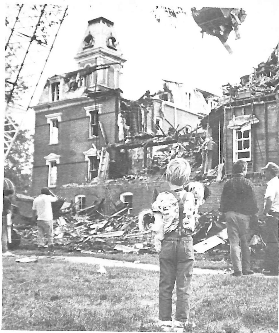
A crane lifts off debris in an effort to salvage faculty files and records. Photo by John Christensen '54.
