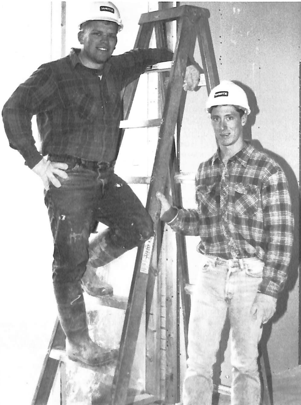
Students in hardhats: Freshmen Nathan Larsen (left) and Darren Tooley are helping build the Old Main replacement.
