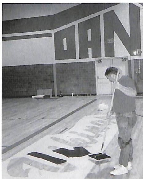
WET PAINT: The gym floor has been resurfaced and repainted as part of the Borup renovation.
