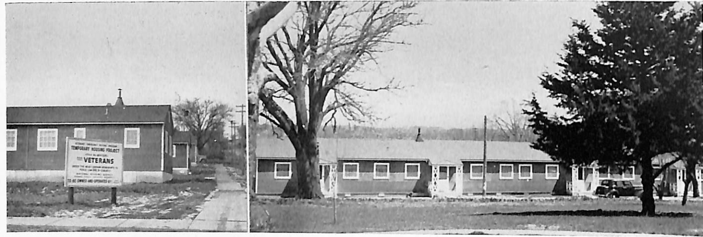
Ten apartments were constructed for veteran families
