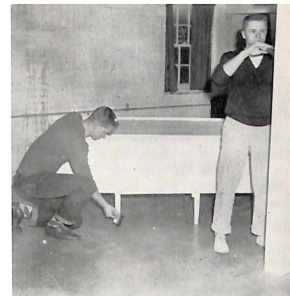
Morgensen and Thomsen apply a coat of paint to the "rec" room and accessories.
