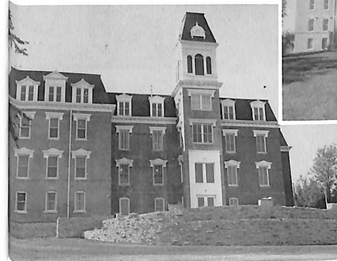
Old Main — before and after
