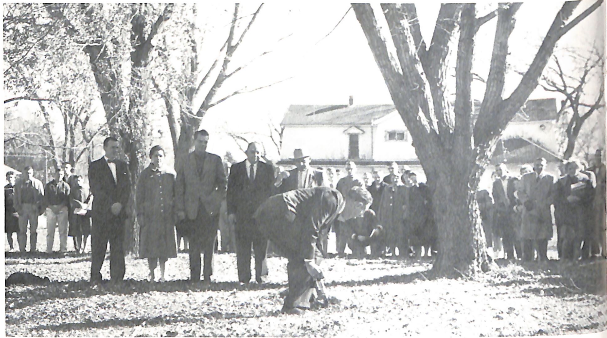
Groundbreaking ceremonies were held for the Charles A. Dana Hall of Science on November 8, 1961.
