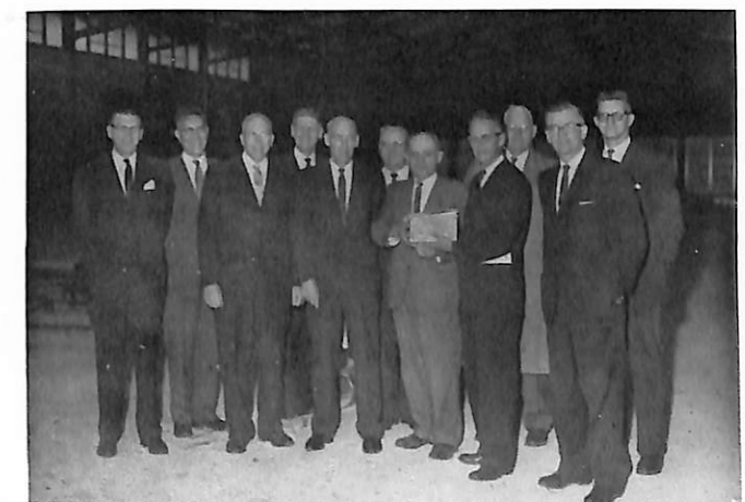
The cornerstone was laid for the Borup Memorial Physical Education Building.
