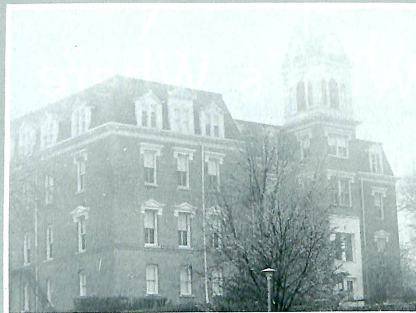
Occupying space on the Dana Campus is Old Main, which has undergone many changes since 1886. Only the middle part is the original building — additions to both and the north give it its present appearance. Plans are presently underway to renovate this historical building.
