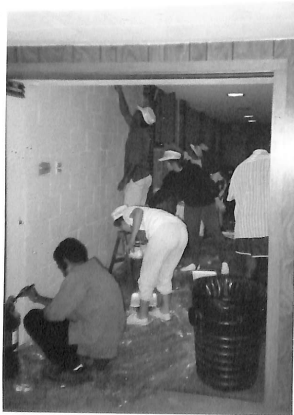
Campus Ministry helped repaint a church down in Lincoln, Ne.
