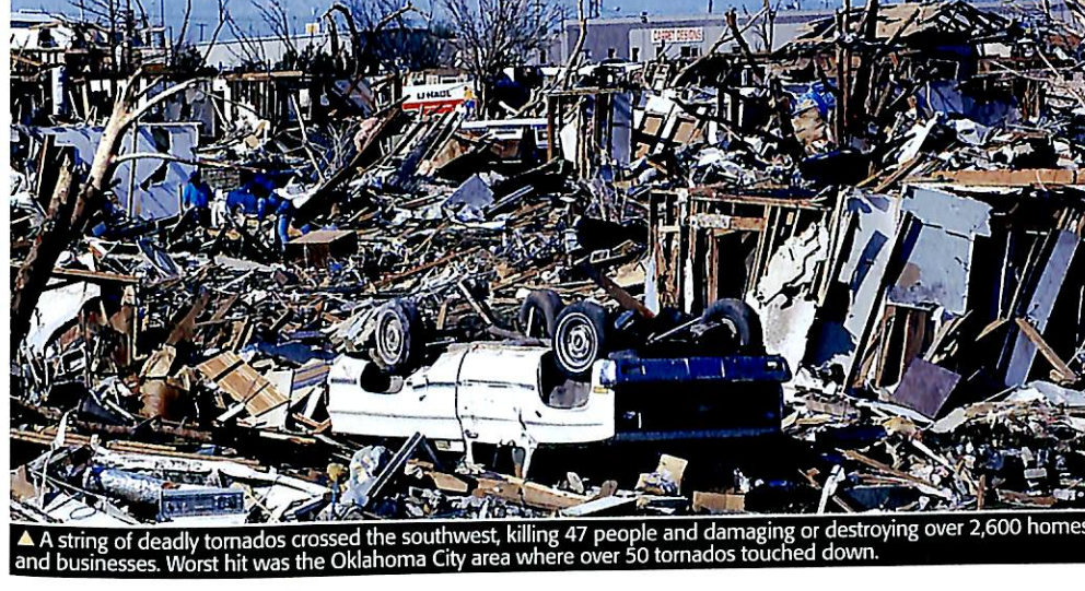
▲ A string of deadly tornados crossed the southwest, killing 47 people and damaging or destroying over 2,600 homes and businesses. Worst hit was the Oklahoma City area where over 50 tornados touched down.
