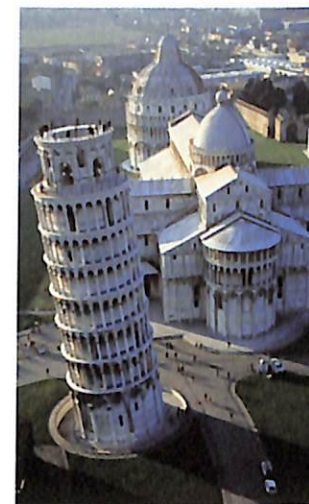
After 12 years of construction, the efforts to stabilize the Leaning Tower of Pisa are complete.
