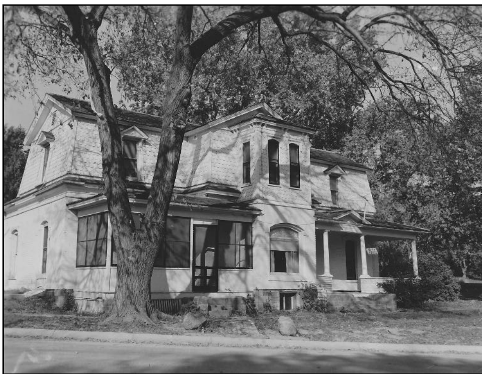
The east-facing Kline House wasn't always painted white. A granddaughter recalls cream-colored brick with designs of red brick at the corners and on the walls.
