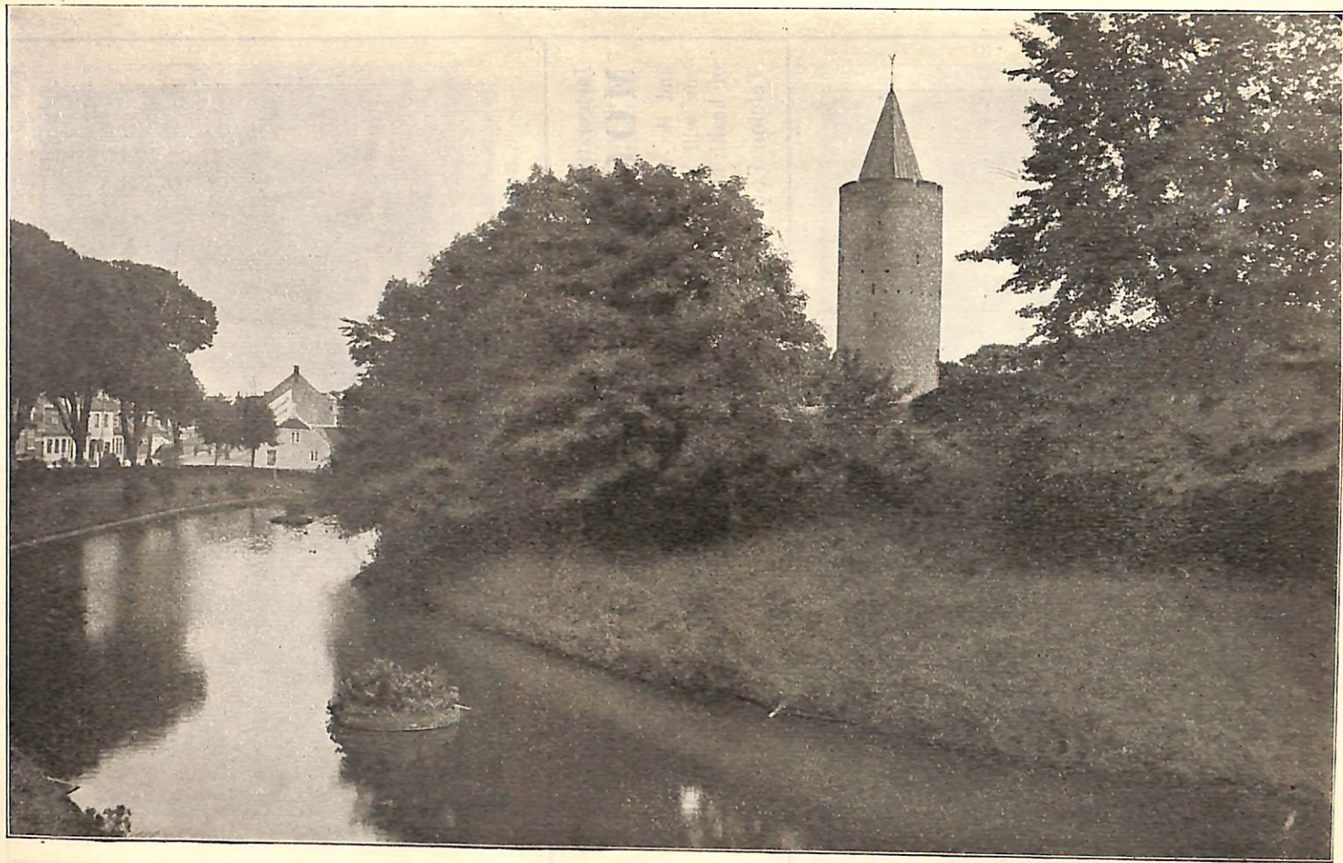
The "goostower" in Vordingborg.
