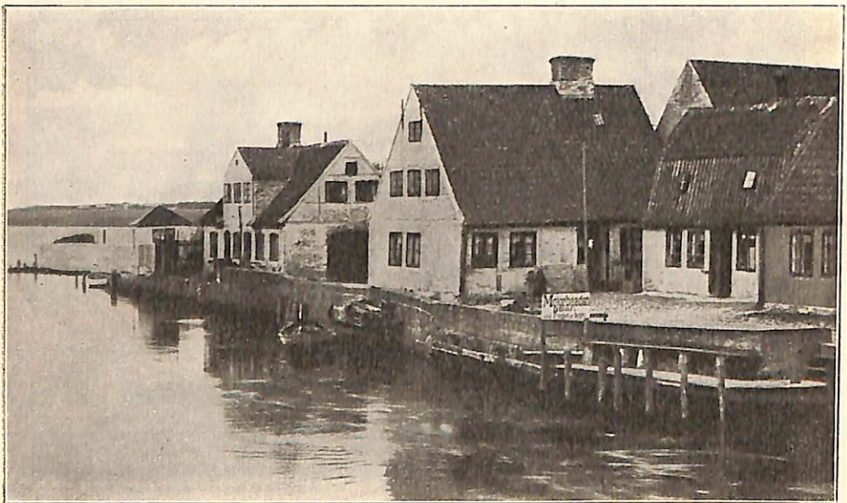
The old bridge in Skelskør harbour.
