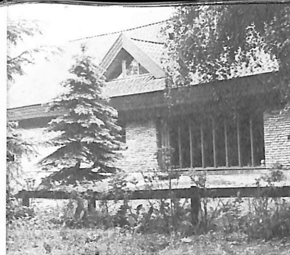
A new house south of Copenhagen reflects the popular trend of blending wood, brick and tile in new house construction.
