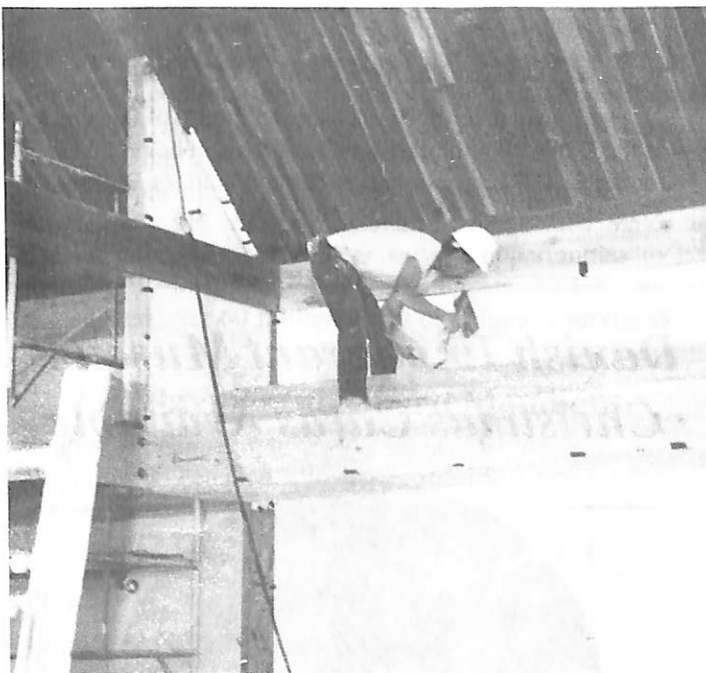
Construction continues on the interior of the Museum.
